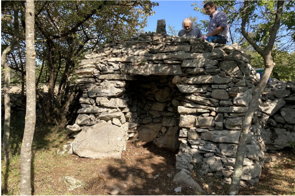
Fig. 6: Completion of the renovation of a demolished stone shelter (hiška). Photo credits: Darja Kranjc
